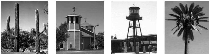
Fig. 2. Base stations are erected on top of many different objects.
