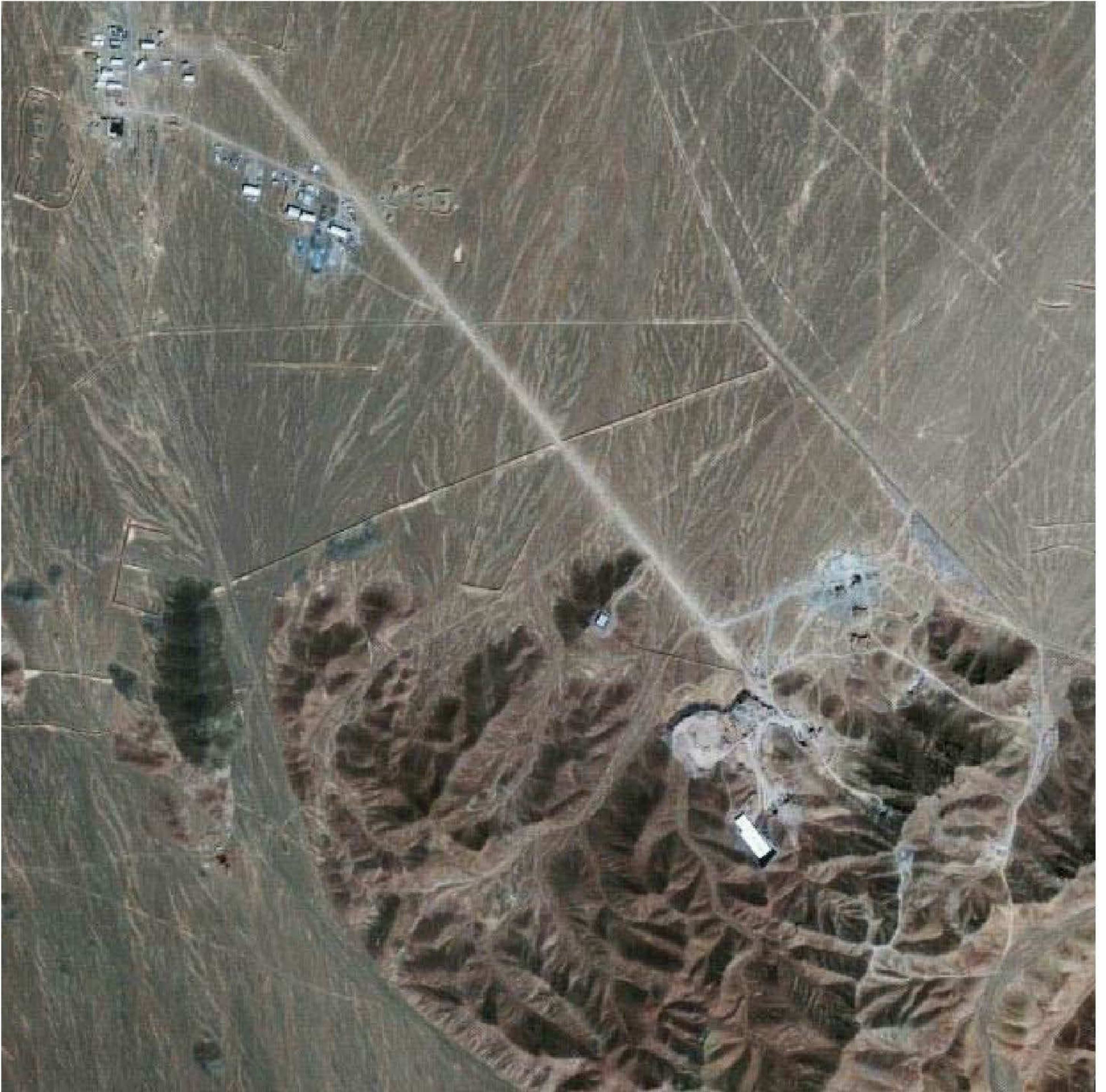
Iran's secret uranium enrichment facility at Qom; tunneling at the site was first revealed by the NCRI in 2005. Photo Credit: GeoEye
