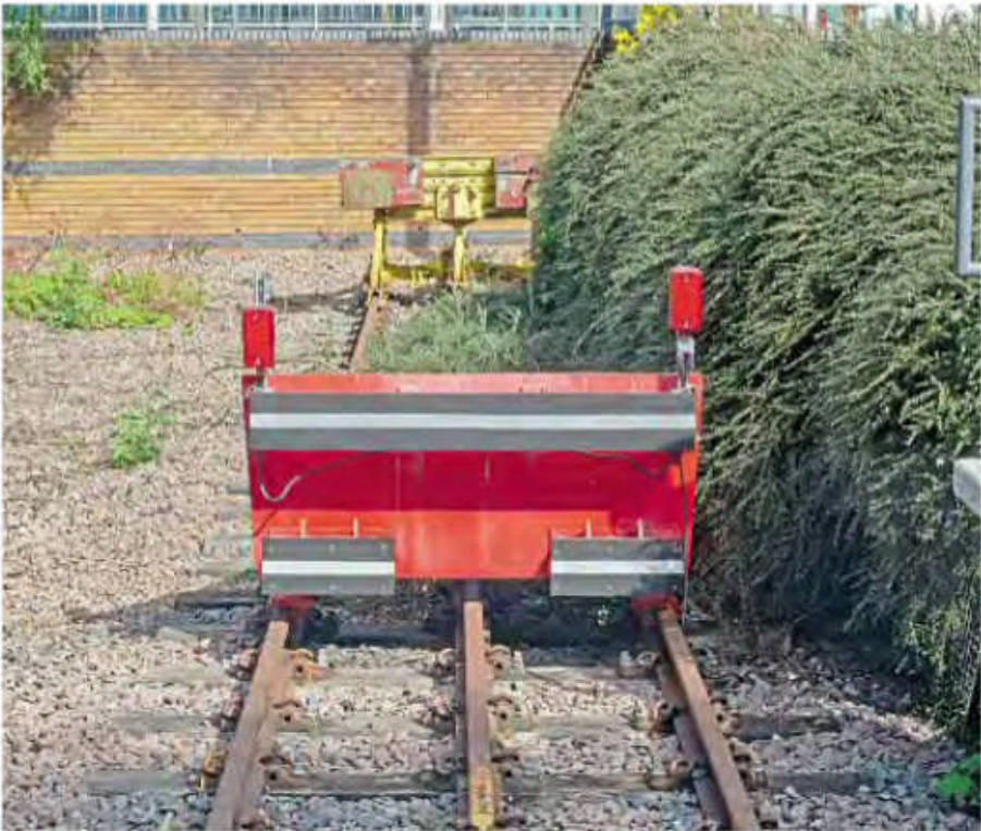
Because of the light construction of the Class 139s, special buffer stops were fabricated as conventional ones would cause considerable damage to the unit. PHIL TONKS
